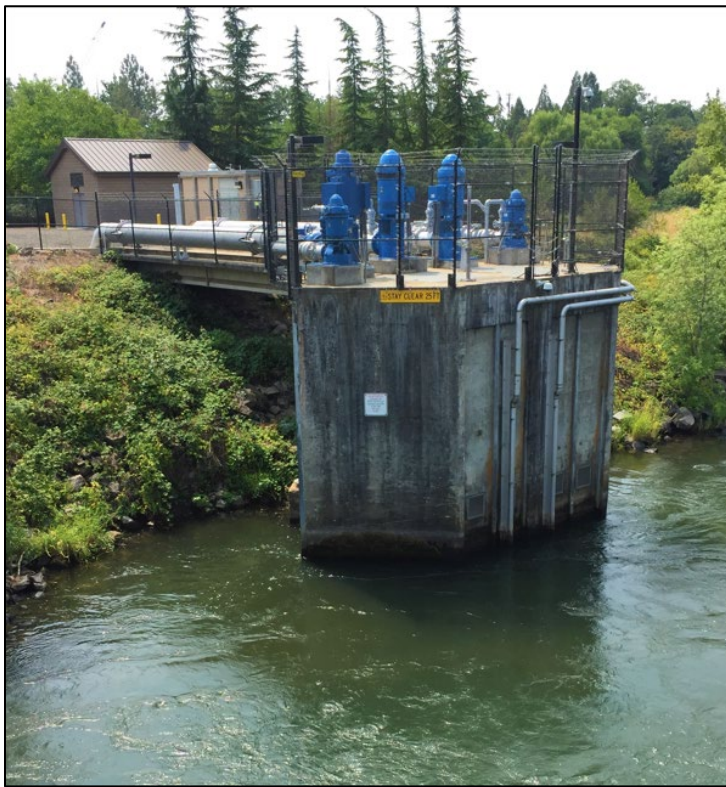
FIGURE 9. DUFF WTP INTAKE ON THE ROGUE RIVER
