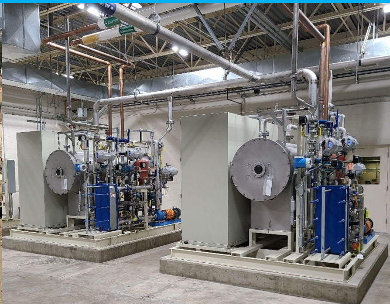
Duff Water Treatment Plant Ozone Generator
