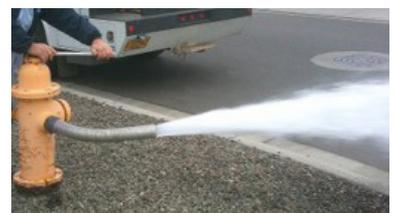
Routine maintenance such as hydrant flushing (pictured above) and valve exercising helps ensure water quality from the source to your tap.
