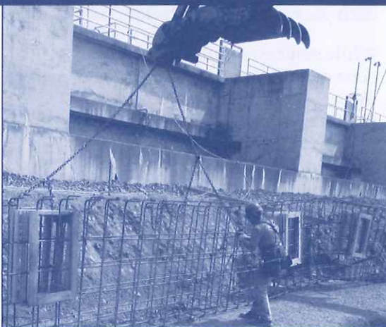
Construction at the water treatment plant
